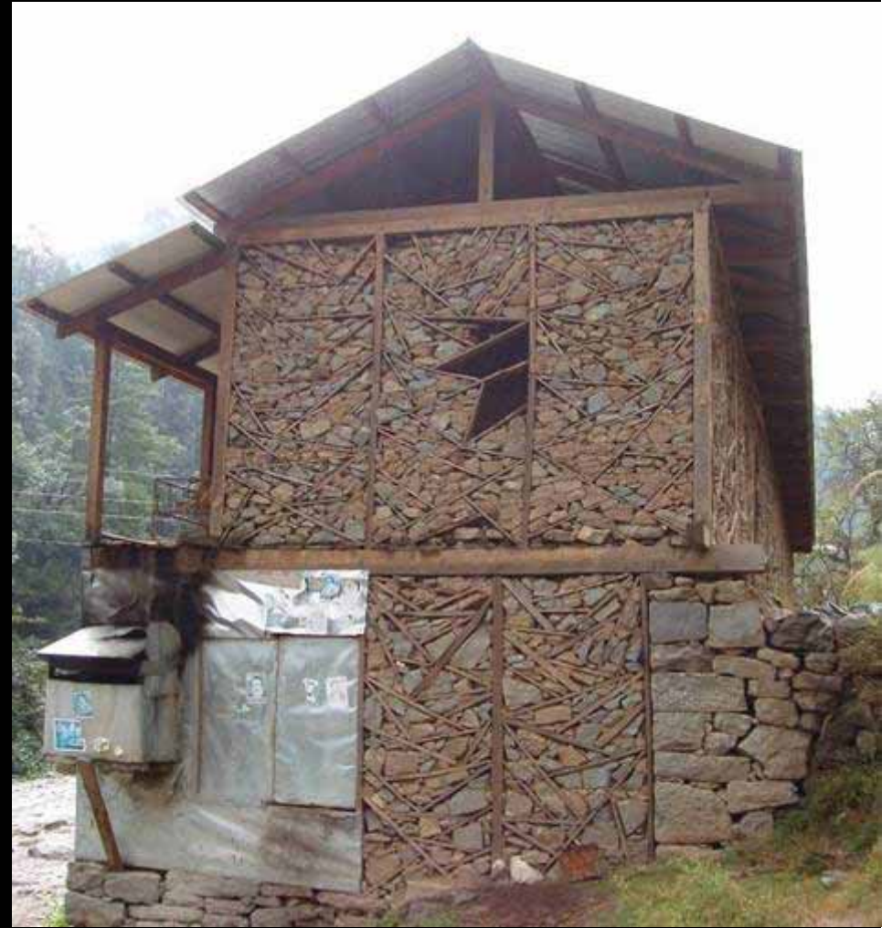
Traditional EQ-resistant dhajji construction in Kashmir
