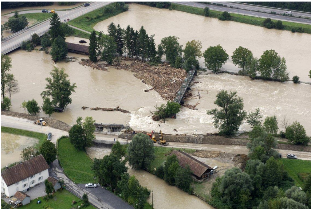
Figure 1: Driftwood accumulation at Weir Perlen during 2005 Flood event (Photo: Swiss Air Force)
