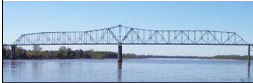
Figure 5: Chester bridge - Illinois
