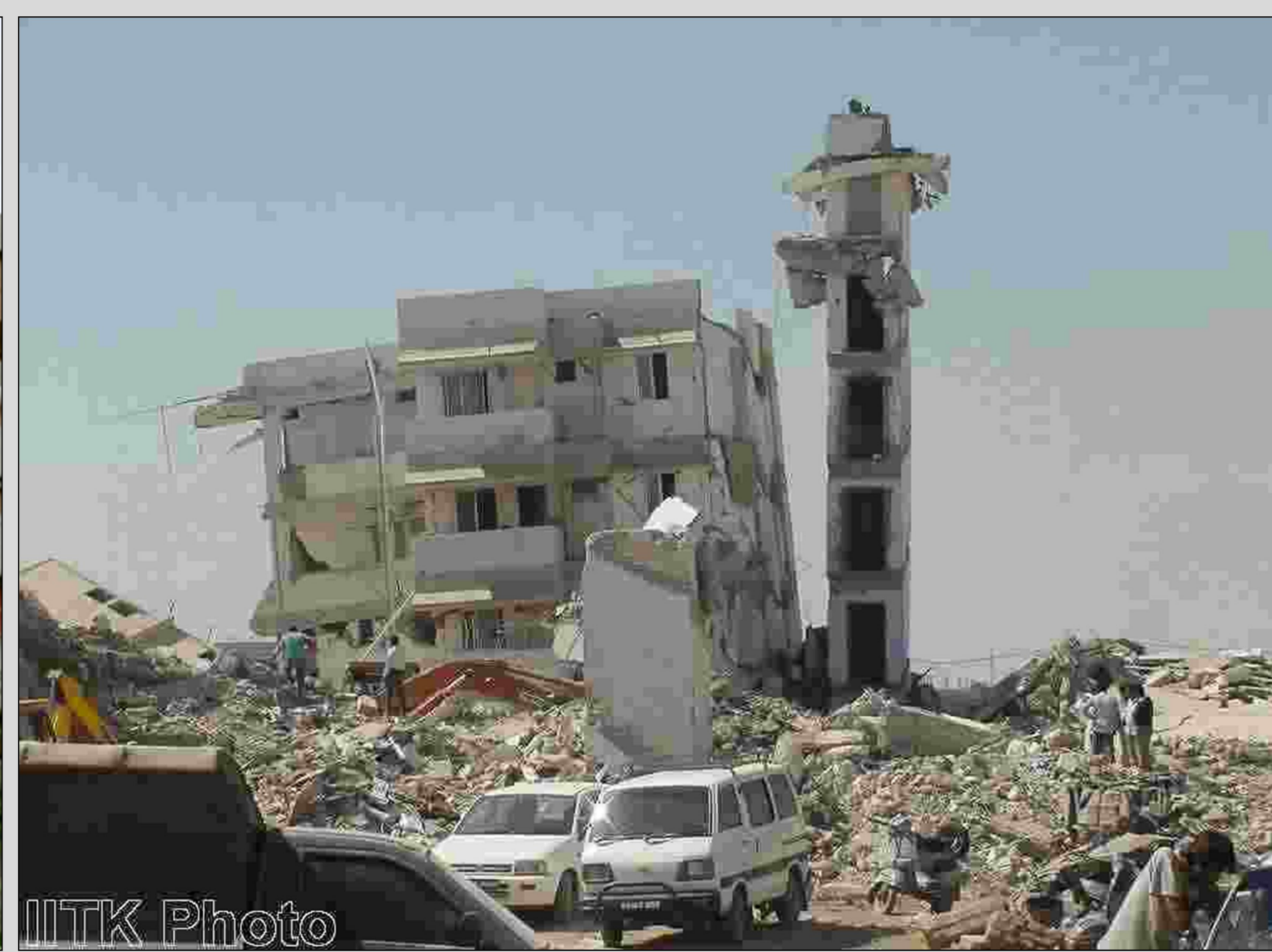
Fig.2 Bhuj, India –Structure with RC core after the 2001 Gujarat Earthquake (R.2.)
