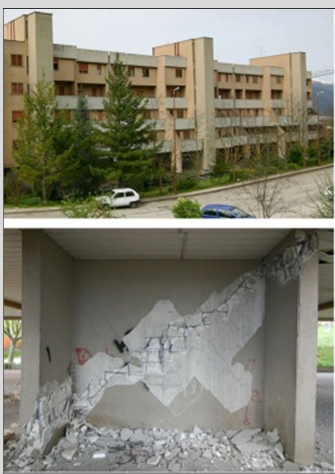
Fig.1 L'Aquila, Italy –2009 Earthquake – RC core wall damage (R.1.)
