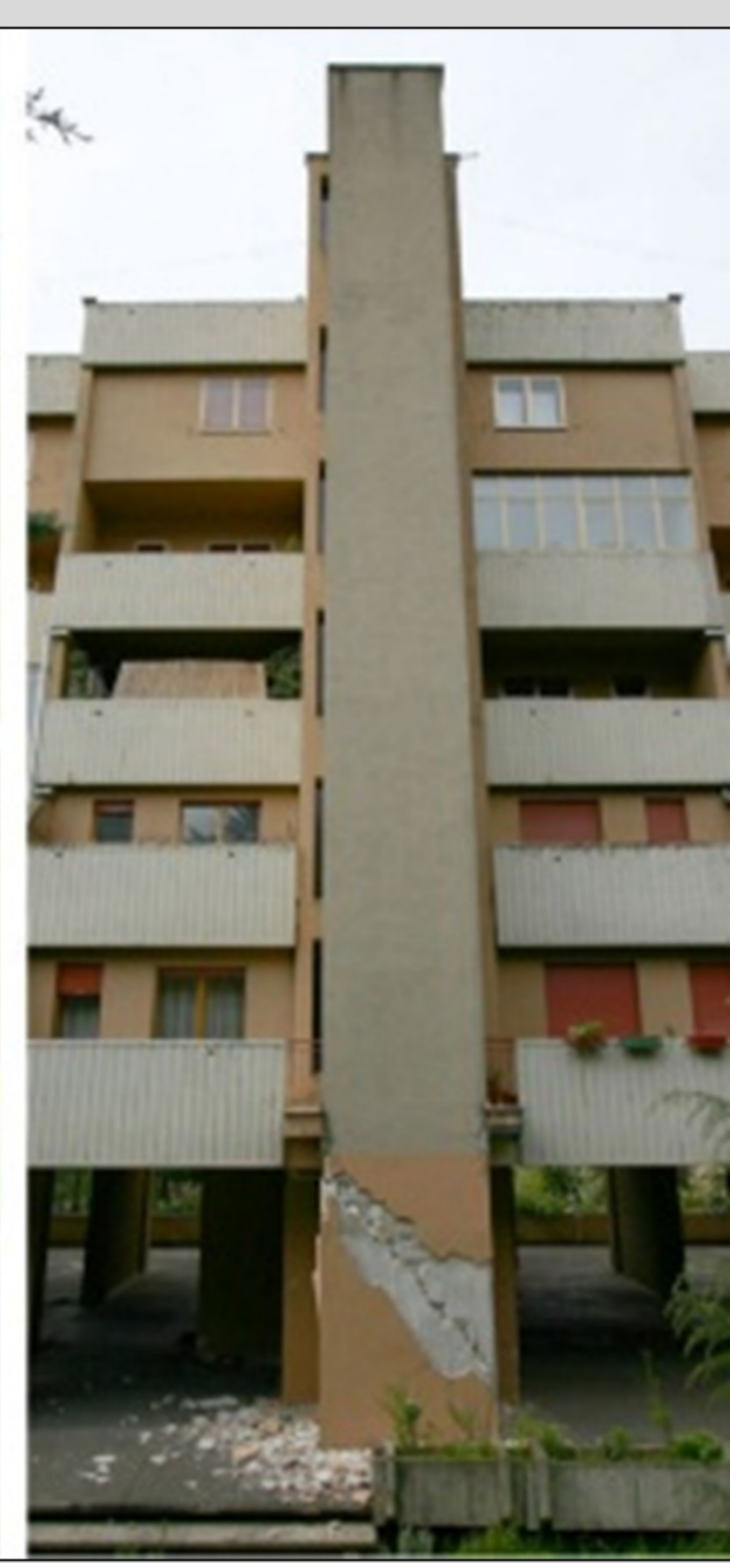
Fig.1 L'Aquila, Italy –2009 Earthquake – RC core wall damage (R.1.)
